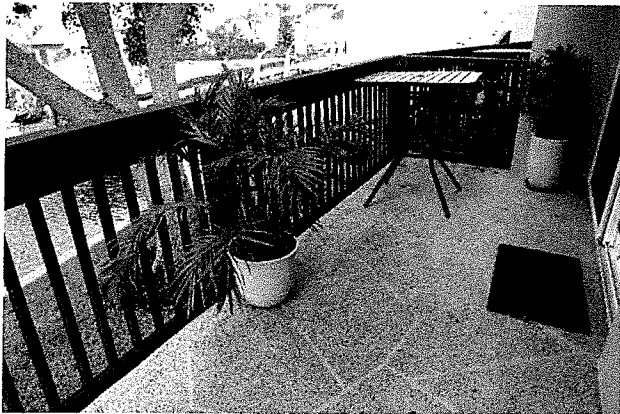
P 67: 2 nd Floor Balcony, Unit 29
