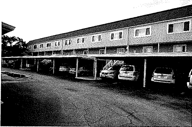
P 1: Elevation, South Building
