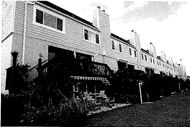
P 11: Rear Elevation, North Building
