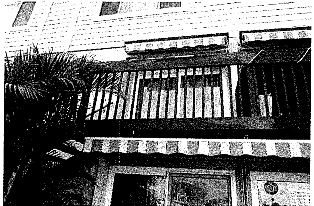
P 16: Deteriorating Wood Railing, West Elevation
