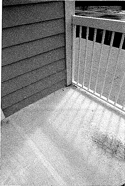
P 61: 3 rd Floor Balcony; Front, Unit 36
