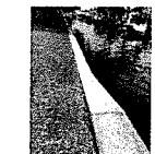
P110 SOUTH SEAWALL
