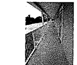
P101 SOUTH BUILDING ELEVATED WALKWAY, AT WESTSIDE FACING EAST
