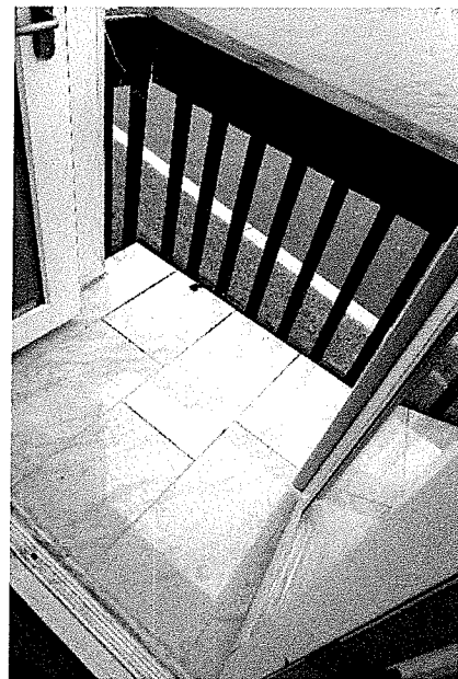
P 60: 3 rd Floor Balcony; Rear Unit 36
