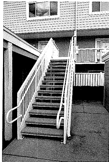
P 4: Stairwell & Gutter Drain
