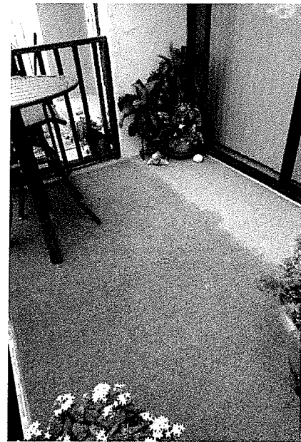
P 76: 2 nd Floor Balcony, Unit 39
