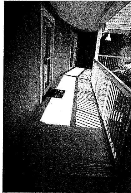
P 94: North Building Elevated Walkway, at Elevator
