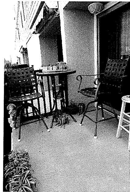
P 80: 2 nd Floor Balcony, Unit 41
