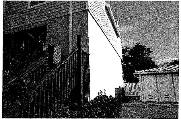
P 34: South Elevation; South Building, Southeast Corner
