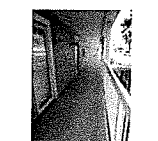
P109 SOUTH BUILDING WALKWAY, AT EASTSIDE FACING WEST
