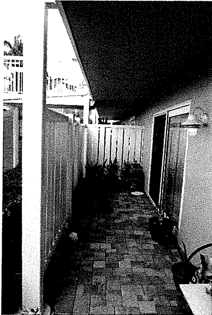
P 7: First Floor Patio
