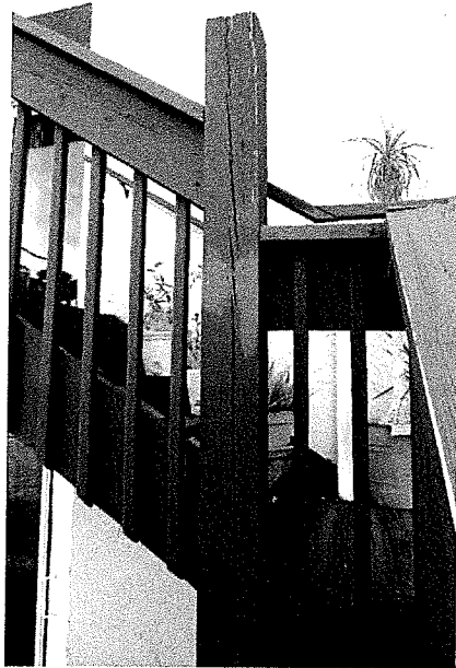
P 17: Split Post, West Elevation
