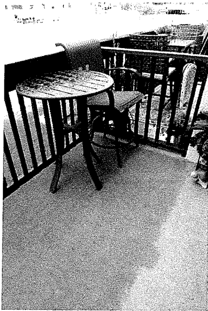
P 77: 2 nd Floor Balcony, Unit 39
