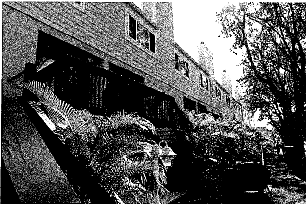
P 31: South Elevation; South Building, Southwest Corner
