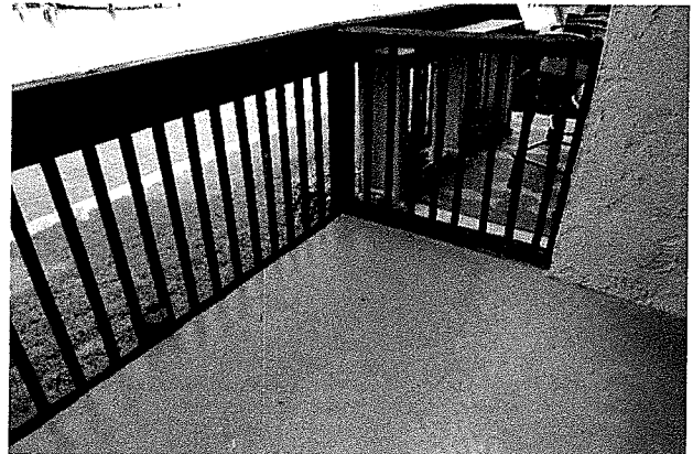
P 72: 2 nd Floor Balcony, Unit 37
