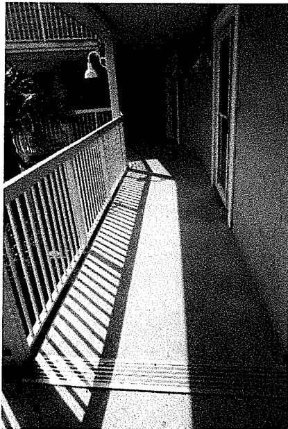
P 95: South Building Elevated Walkway, at Elevator
