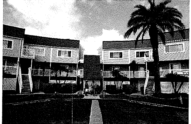
P 2: Elevation, Center
