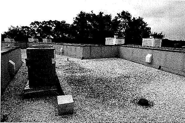
P 51: South Building Roof, at Northwest Corner
