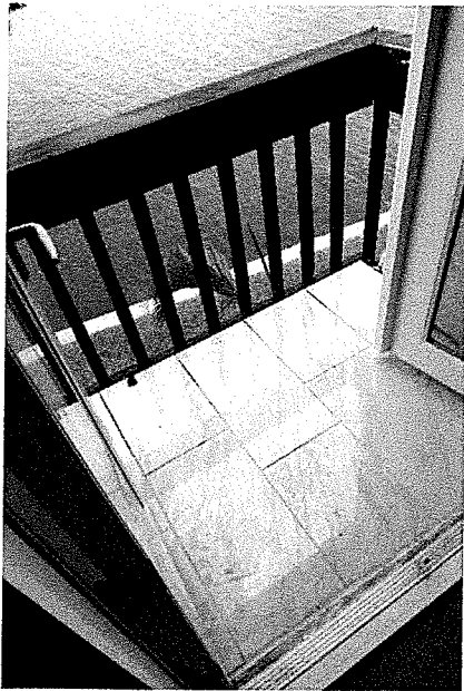
P 59: 3 rd Floor Balcony; Rear, Unit 36
