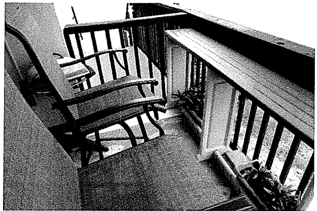
P 74: 2 nd Floor Balcony, Unit 38
