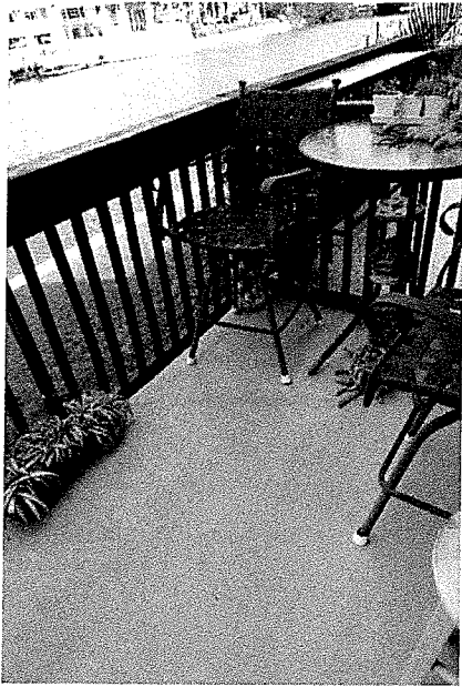
P 81: 2 nd Floor Balcony, Unit 41
