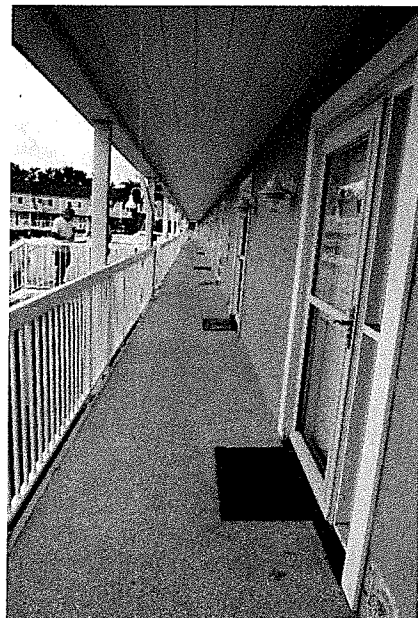
P 84: Elevated Walkway; North Building, at Northside facing South
