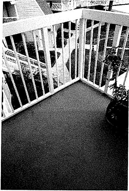
P 65: 3 rd Floor Balcony; Front, Unit 29
