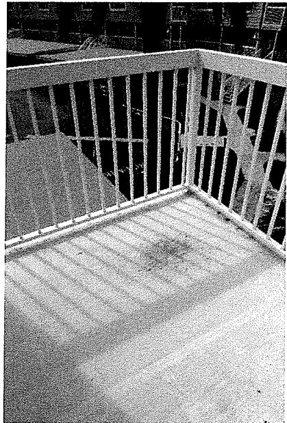
P 62: 3 rd Floor Balcony; Front, Unit 36
