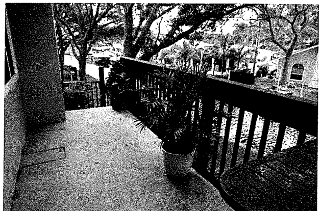
P 68: 2 nd Floor Balcony, Unit 29
