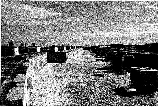
P 45: North Building Roof, at Southside facing North
