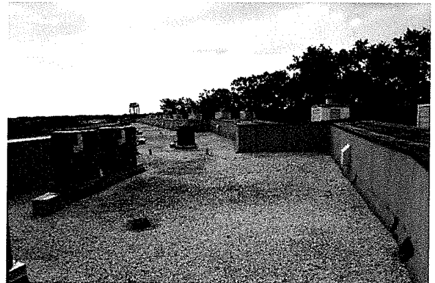
P 52: South Building Roof, at Westside facing Southeast
