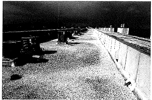
P 46 North Building Roof, at Northside facing South
