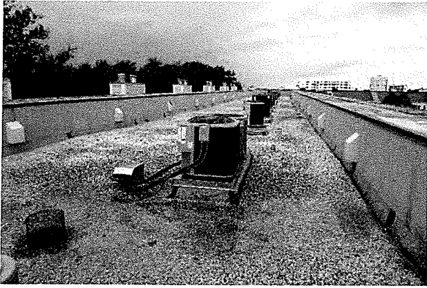
P 57: South Building Roof, A/C Units
