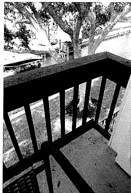
P 64: 3 rd Floor Balcony; Rear, Unit 29
