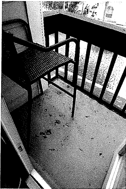
P 63: 3 rd Floor Balcony; Rear, Unit 29
