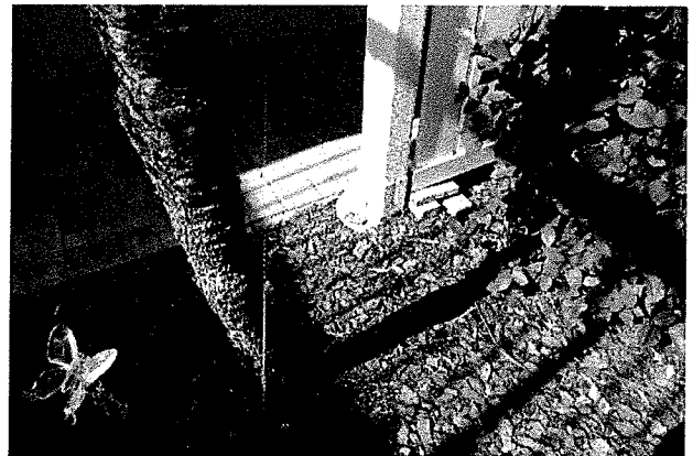
P 38: Rusted Steel Base; North Elevation, South Building
