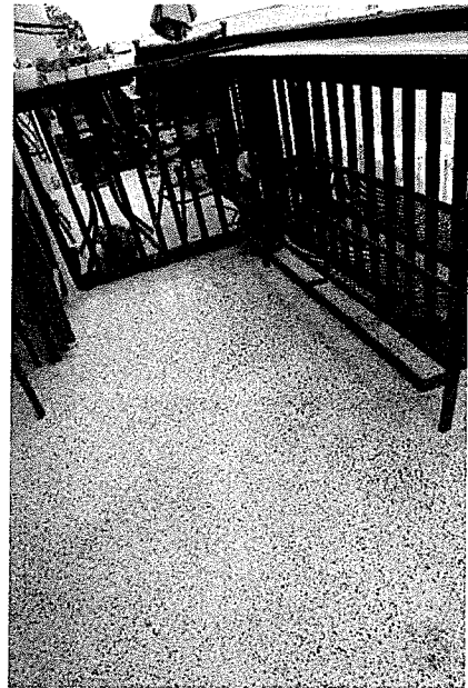
P 82: 2 nd Floor Balcony, Unit 42
